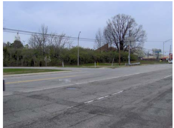
Kenwood & 71 SB heading West
